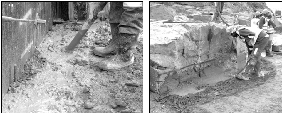
Figure 7. Compaction of 400mm wide GE-RCC strip against formwork and the rockface.
