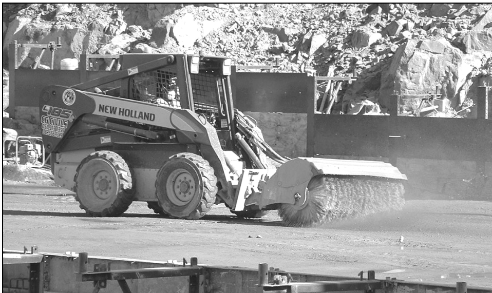
Figure 8. Green cutting of the RCC surface using the Bobcat mechanical broom
