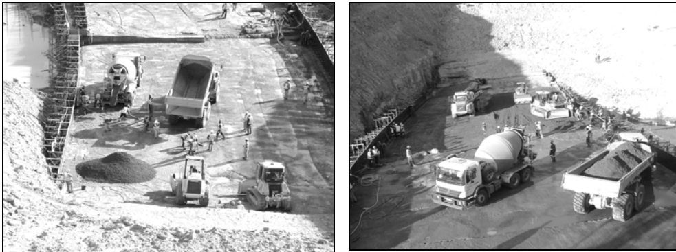
Figure 6. Placing of bedding mortar, dumping of RCC, levelling and compaction thereof.
